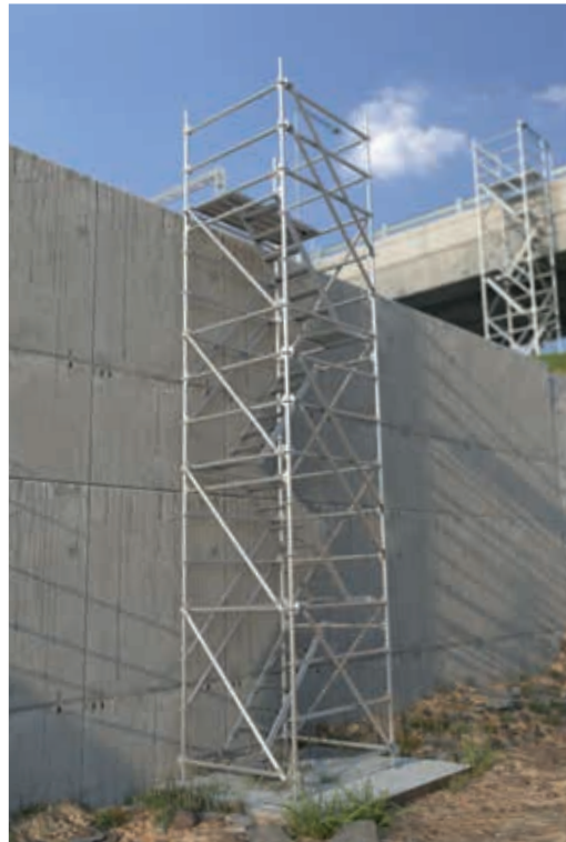
Stair tower site access
